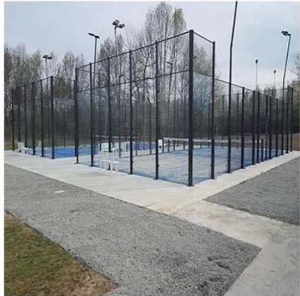
Italy stadium project
