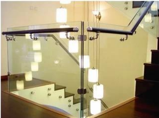
10.76 thick clear laminated glass application:
