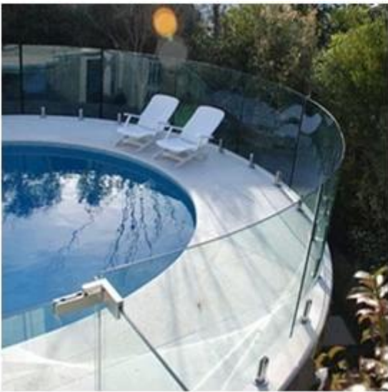
10mm toughened frameless balustrade curved glass.
