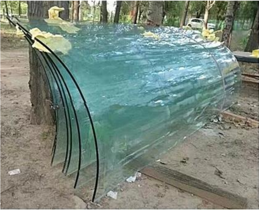
10mm clear curved tempered glass used for handrail.
