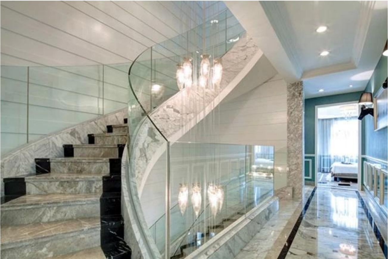
10mm toughened frameless balustrade curved glass.
