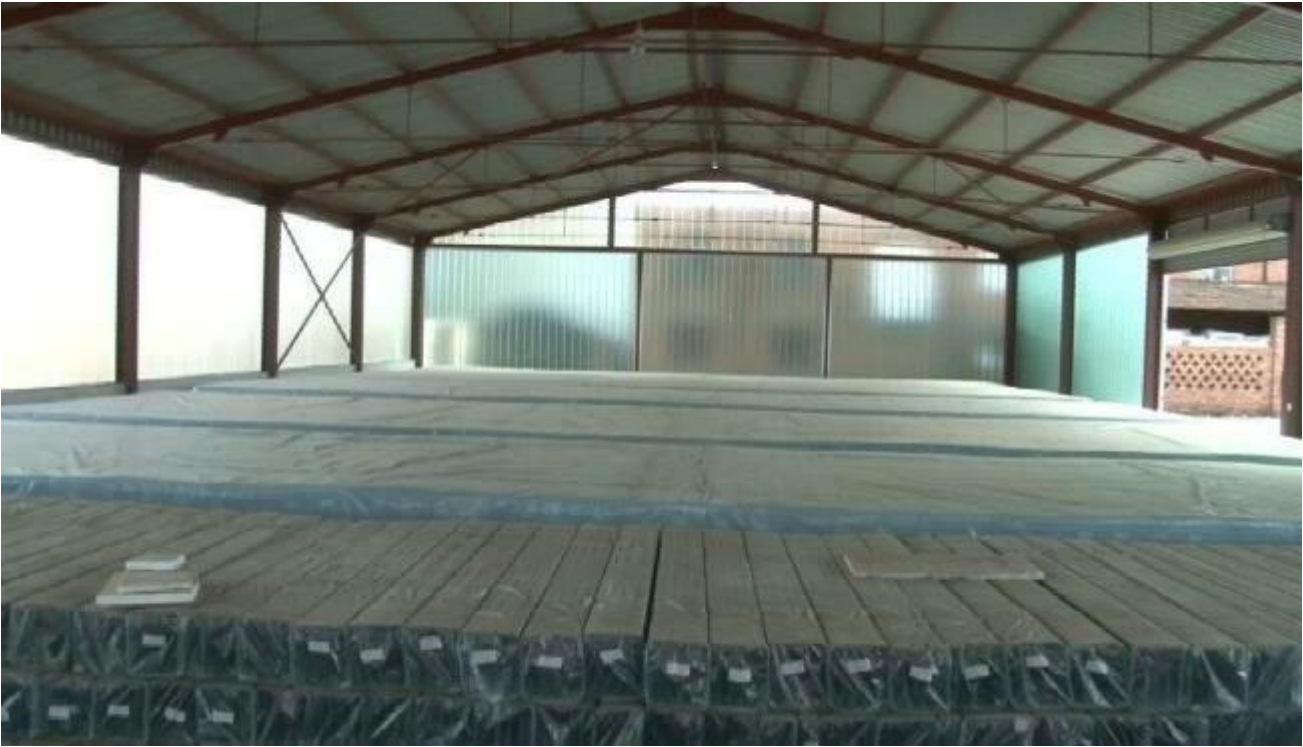
U shaped glass production line by Jimy Glass Factory
