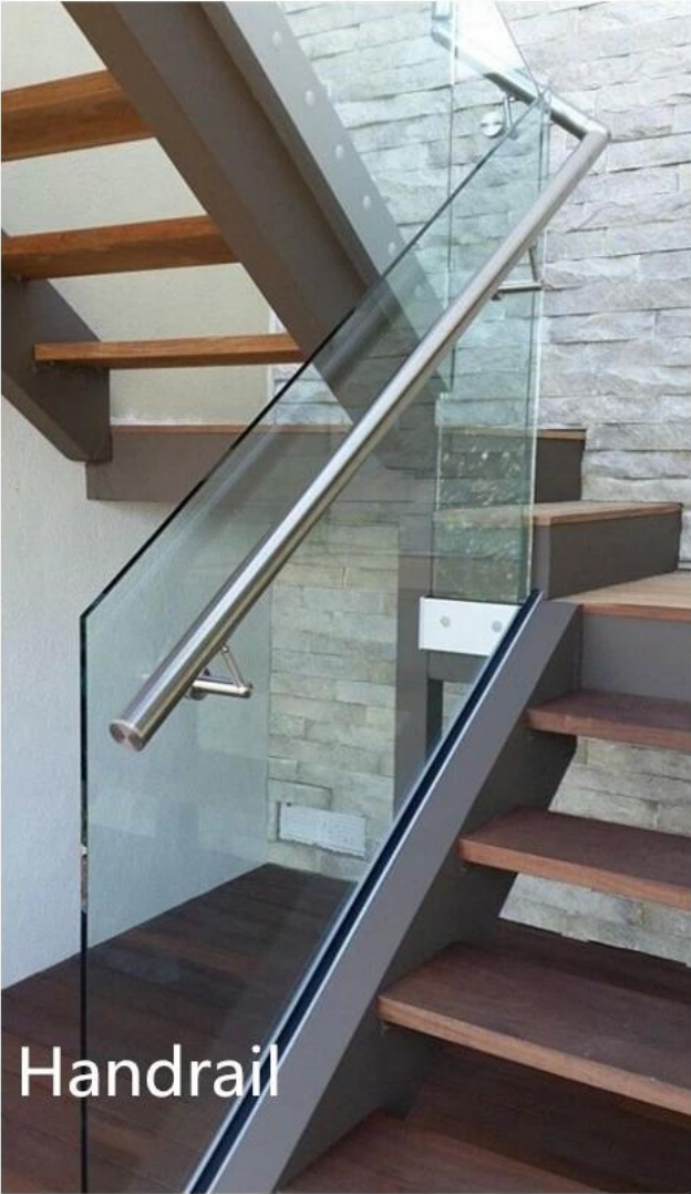
railing with bolt fixing
