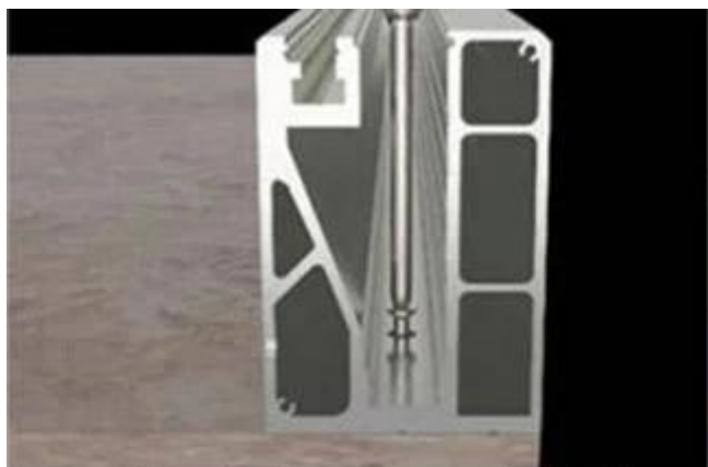
screw the aluminum groove to the floor and drill the drain hole
