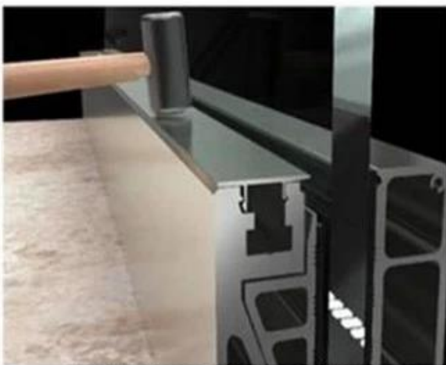
put the top cover over the screw
