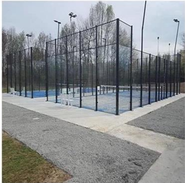
Italy stadium project
