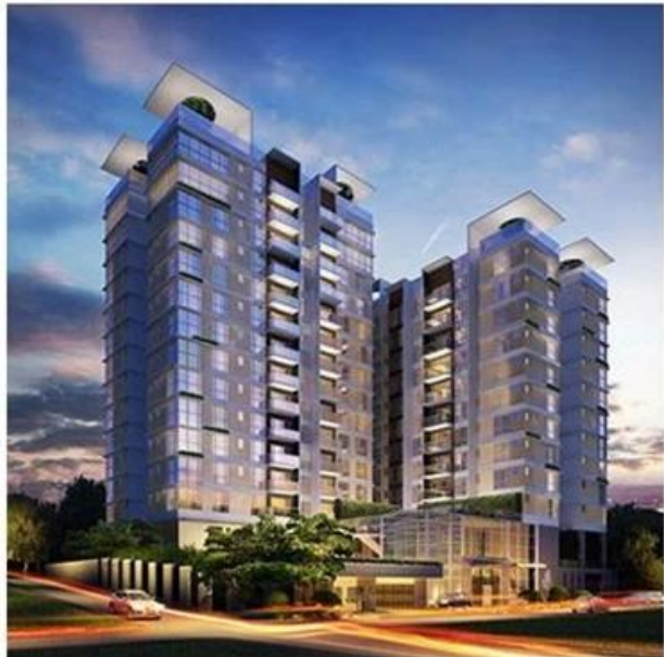
Philippines Facade Project
