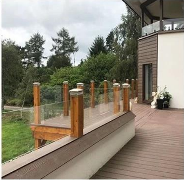
Britain Railing Project
