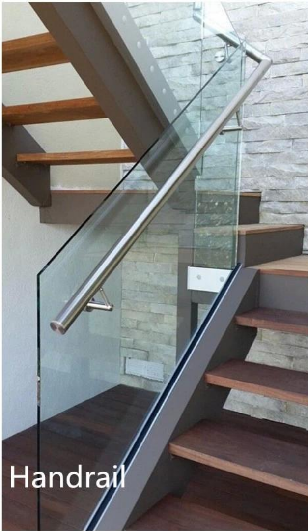
railing with bolt fixing
