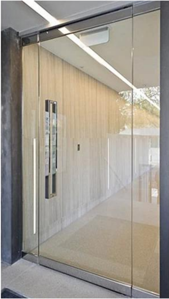
12mm tempered glass for entrance door :
