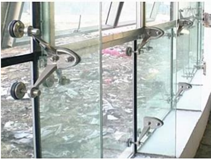
laminated glass facade support fin:
