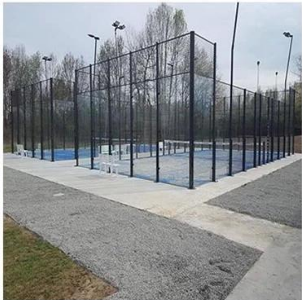
Italy stadium project
