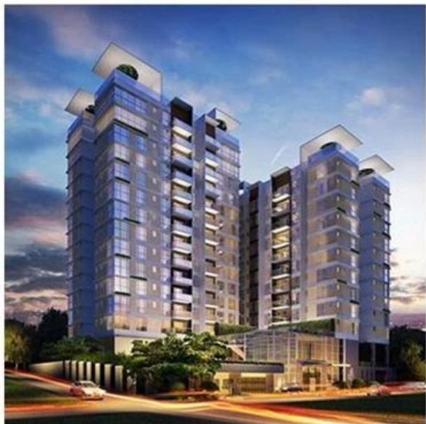
Philippines Facade Project
