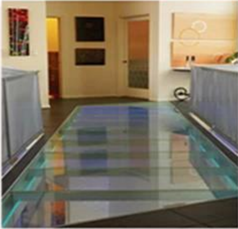
Laminated tempered PVB Film glass application
