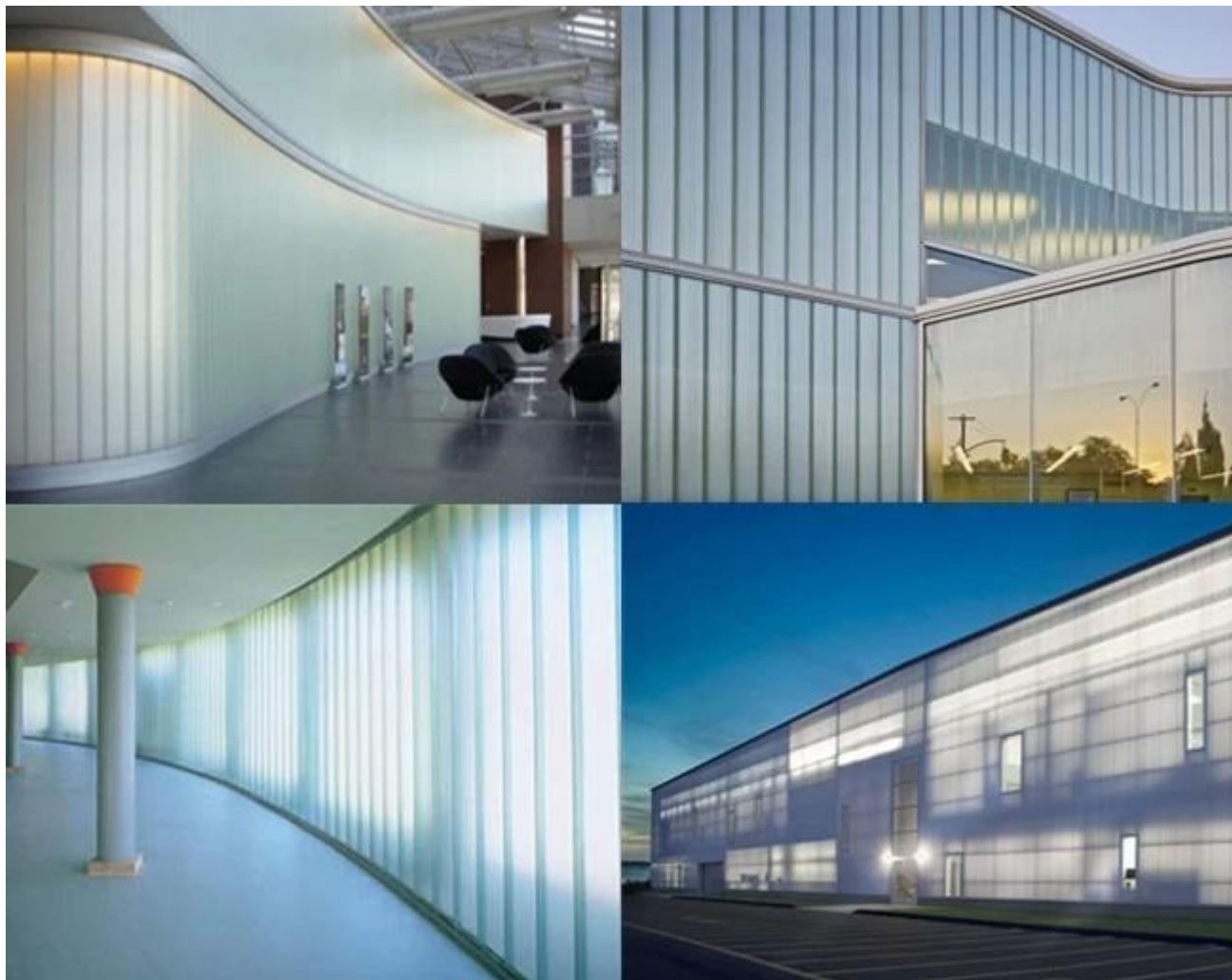
Flat curve low e double glazing unit curtain wall
