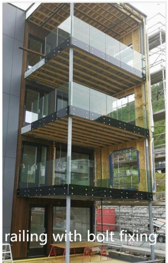
railing with bolt fixing
