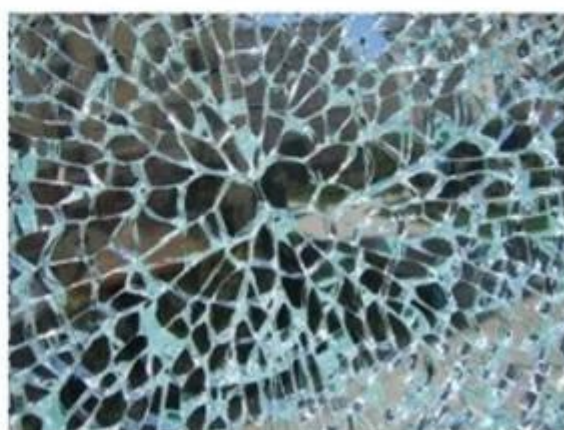
Tempered laminated glass with very strong external force cubical debris will fall down
