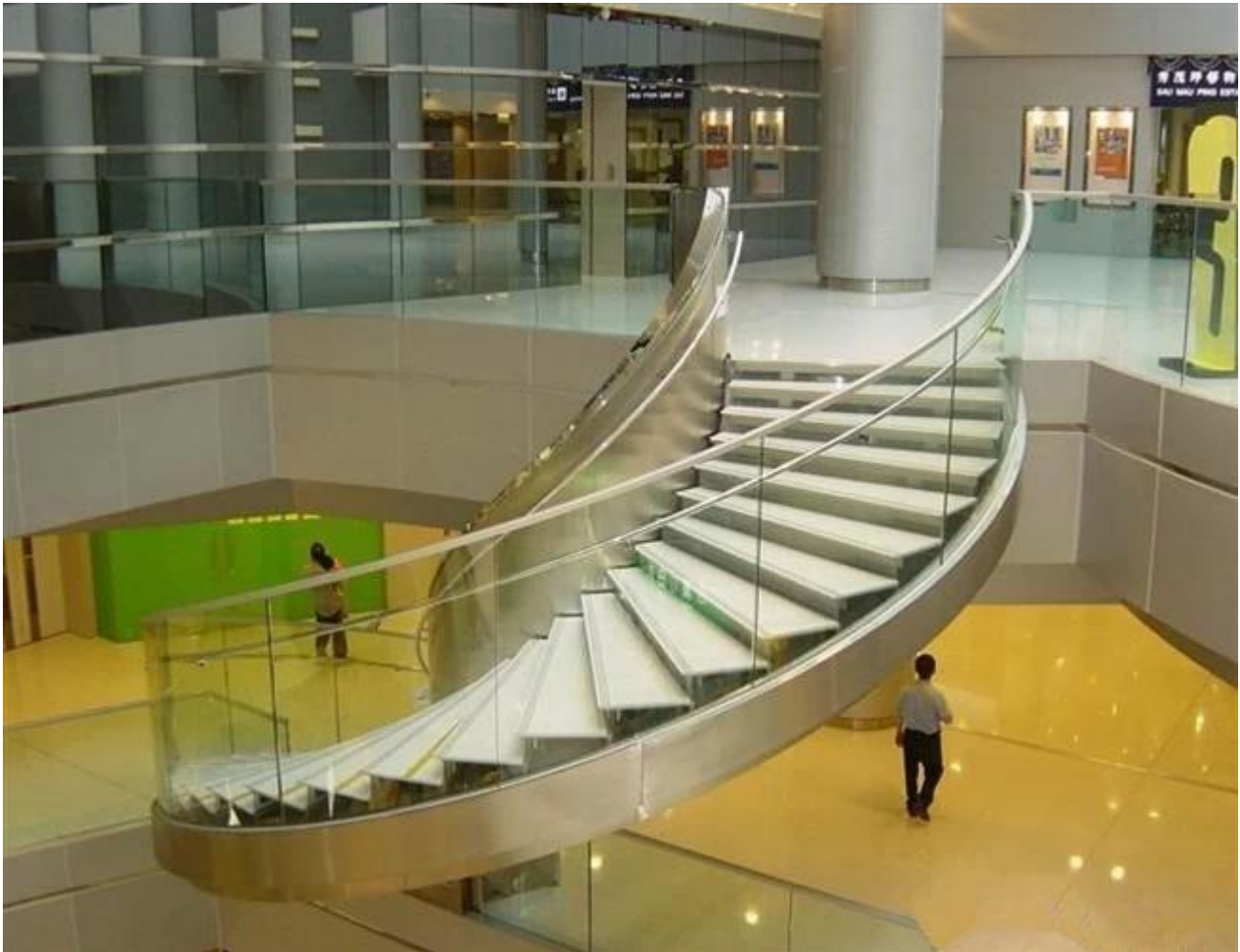
10mm clear curved tempered glass used for handrail.
