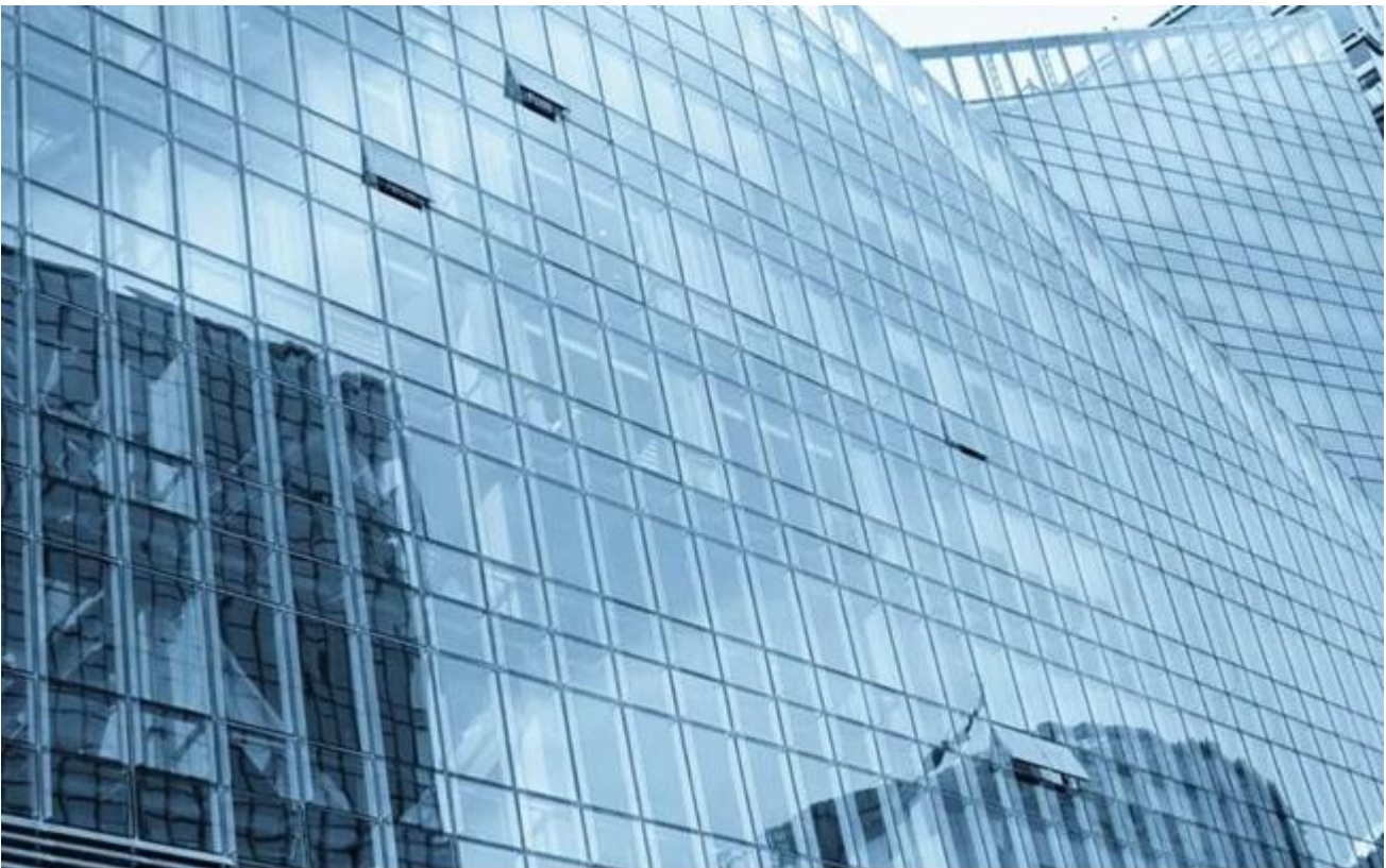
12mm heat-strengthened glass made into laminated glass or insulated glass,use for glass curtain wall and outside glass window in tall building.
