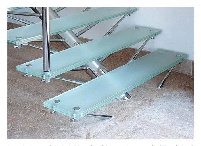
Screen printing decorative laminated glass, it is made from one piece <u>screen printed glass</u> with two pieces clear toughened glass bonded together with colorless PVB or SGP. The screen printing glass, is a kind of anti-slip glass, also a kind of decorative glass, could make the stair more esthetic. We could do full surface color screen printing glass, also could do dot silkscreen glass, line silkscreen glass, etc. The color is variety, select by customers.
