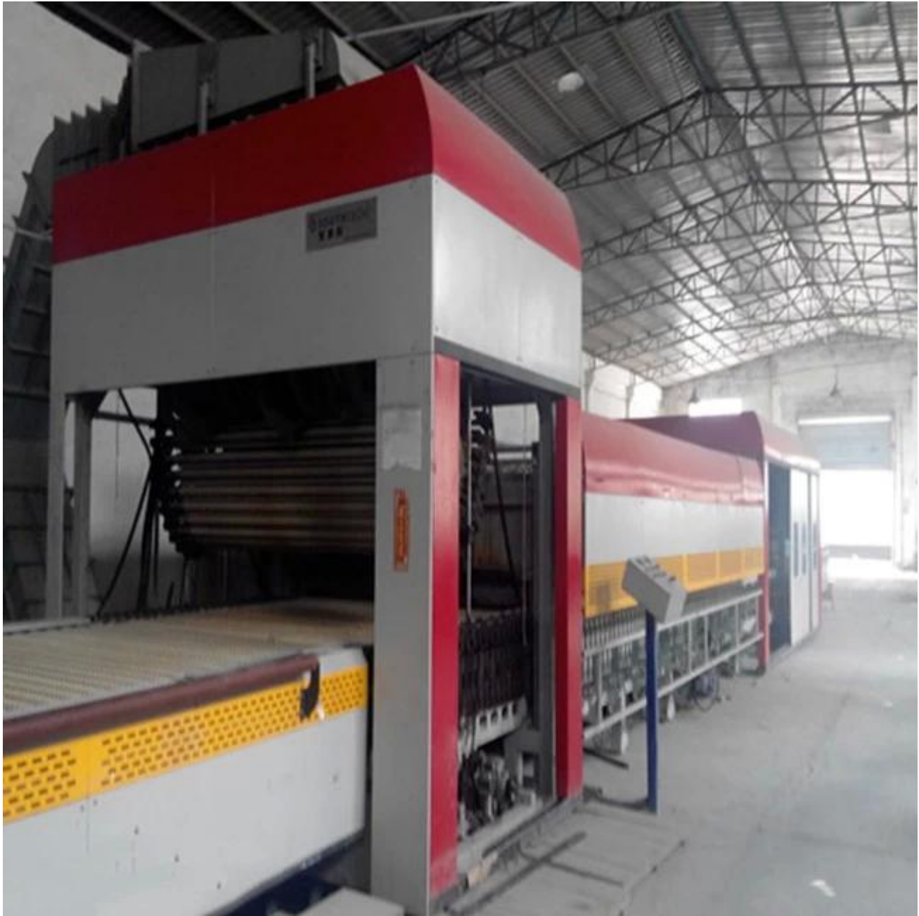
Laminated Glass Production Plant
