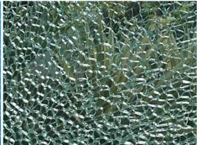
Tempered laminated glass broken
