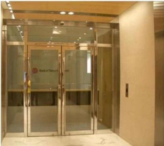
Insulating fire-resistant glass used for buildings partition
