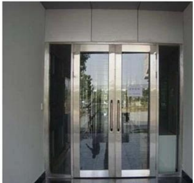
Insulating fire-resistant glass used for buildings partition
