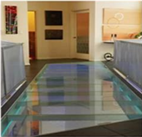
Laminated tempered PVB Film glass application
