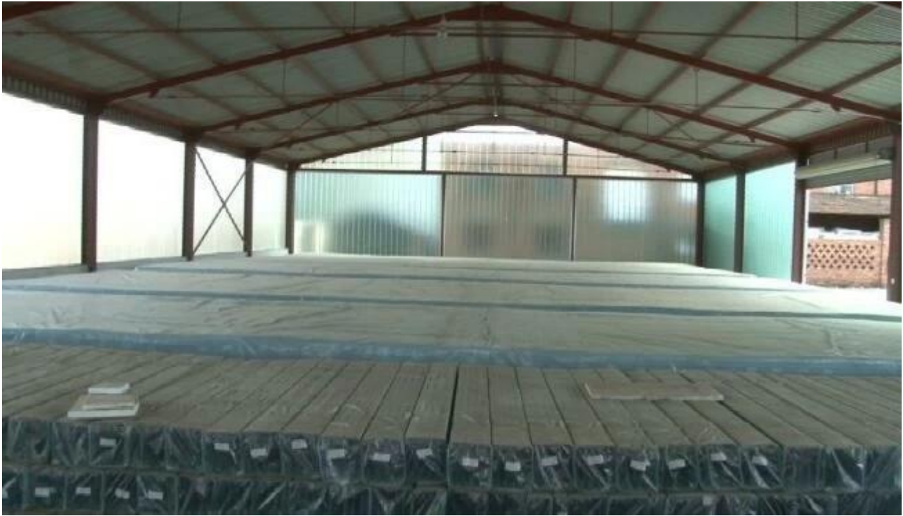
U channel glass production line by Jimy Glass Factory
