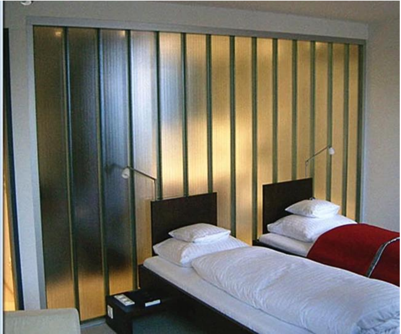
7mm U channel glass curtain wall:
