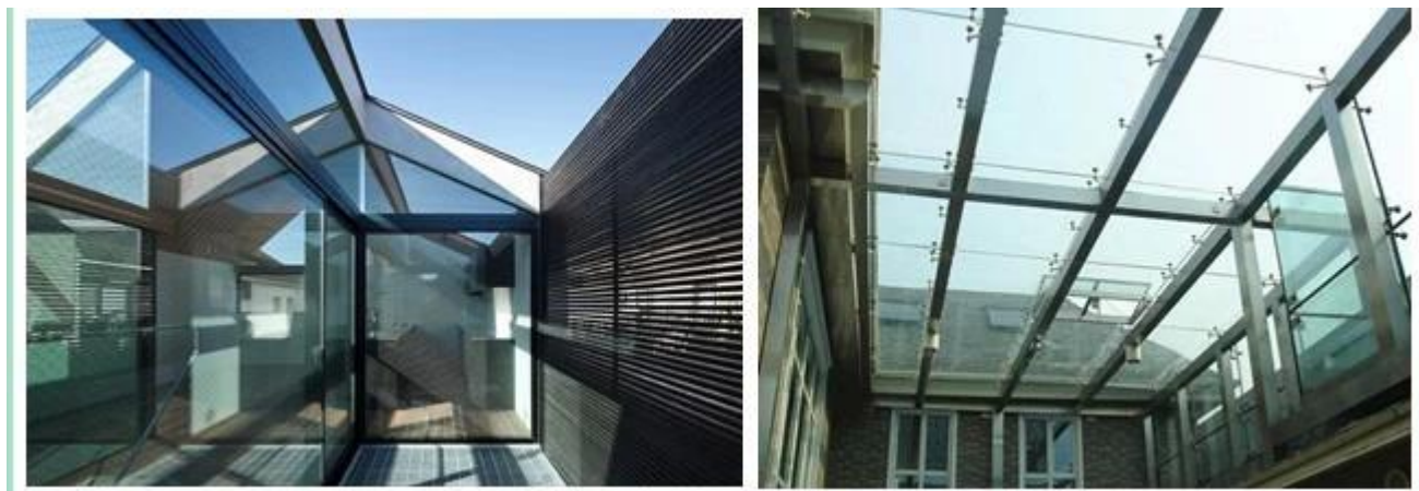
Insulated glass used for skylight:
